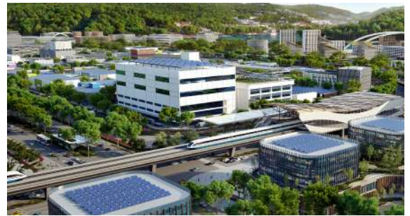
Green Tech Park LRT Station
